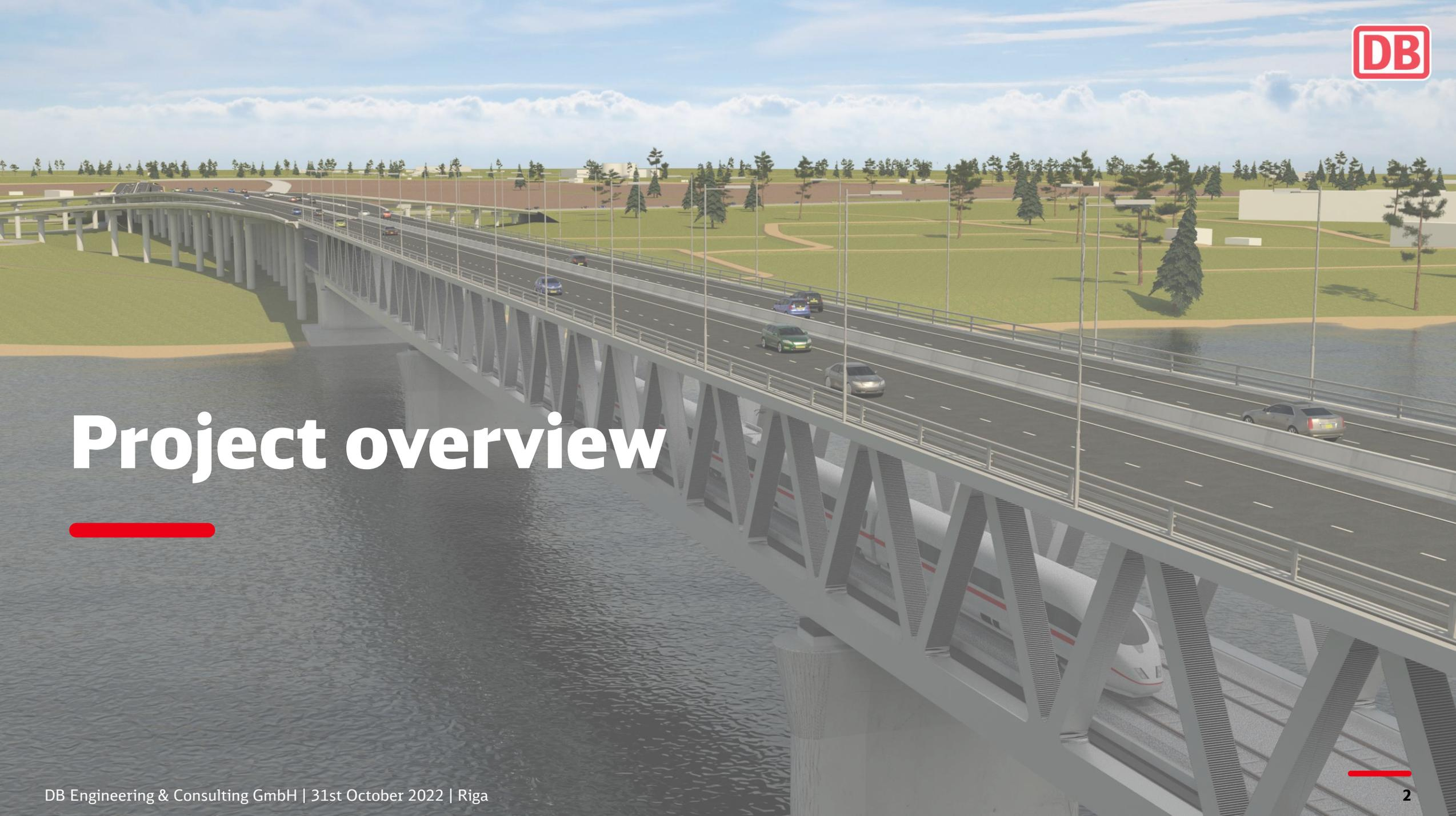
A 3D architectural rendering of a large, multi-level bridge spanning a body of water. The bridge has a complex truss structure. The top level is a highway with several cars. Below it is a railway track with a high-speed train. The bridge is supported by numerous concrete piers. The background shows a green landscape with trees and a blue sky with clouds.
