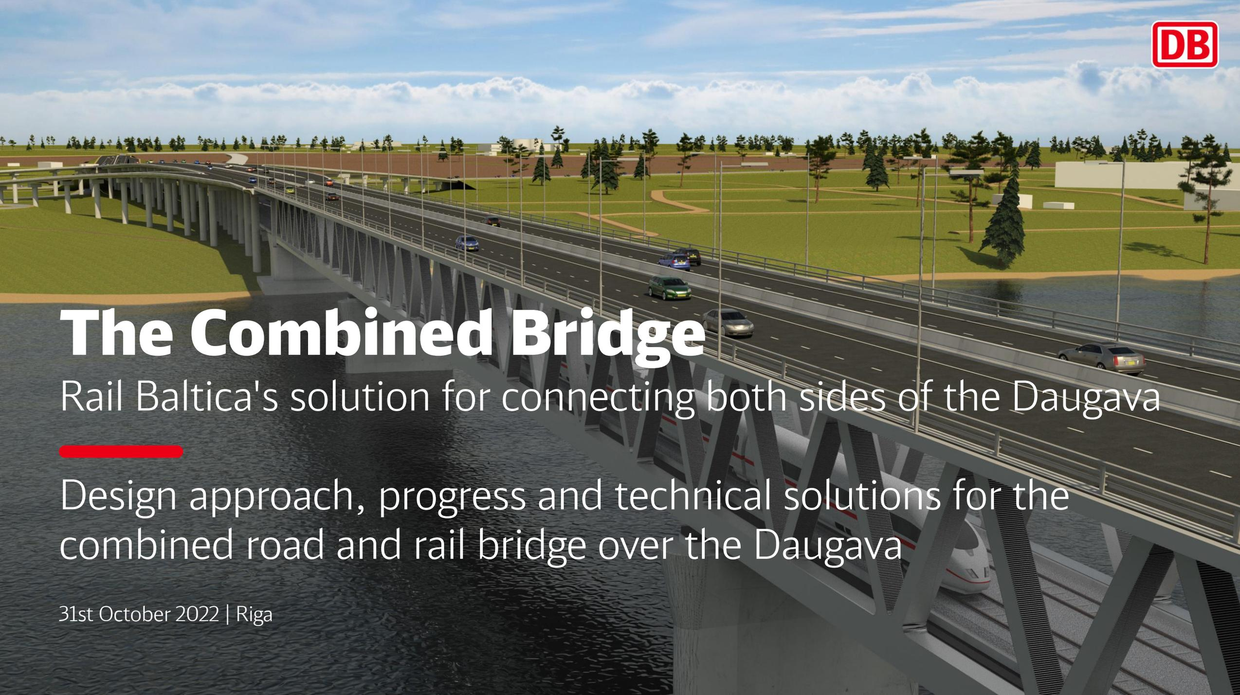
A 3D architectural rendering of a large, modern bridge spanning a wide river. The bridge has a complex steel truss structure. On the upper level, there are multiple lanes of a highway with several cars driving. On the lower level, a high-speed train is visible. The background shows a green landscape with trees and a clear blue sky with some clouds.
